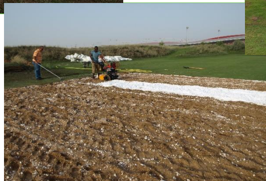
Laying Fytofoam® in an existing grass cover
