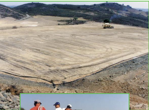
Laying Fytofoam® for a football pitch under extremely dry conditions in Portugal. Viewed anti-clockwise:
