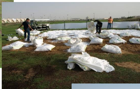
Laying Fytofoam® in an existing grass cover
